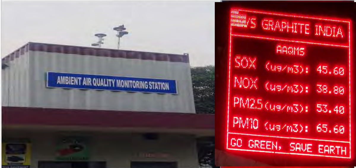
For EC compliance Ambient Air Quality Monitoring Station (AAQMS) with Outside LED Display unit Installed -Commissioning is in process
